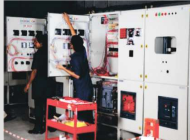
Electrical Wiring of Panels
